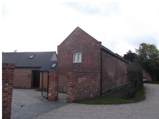
Picture B.6 A further example of localised repointing
