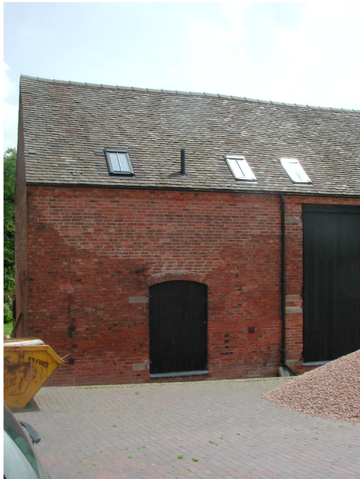
Picture B.8 A further example of a refurbishment which maintains an unbroken roofline
