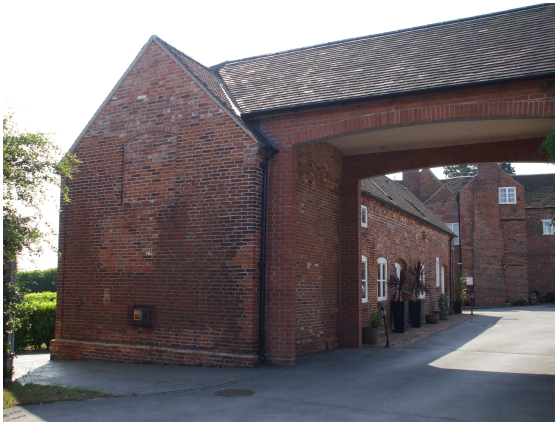
Picture B.7 An example showing how refurbishment should maintain an unbroken roofline
