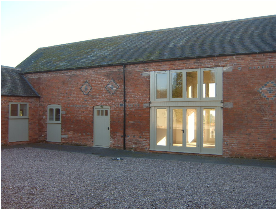
Picture B.3 Example of utilising existing openings to maximise natural, internal light
