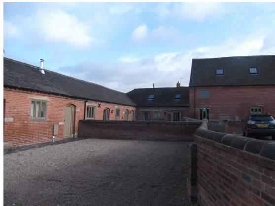
Picture B.5 An example of localised repointing
