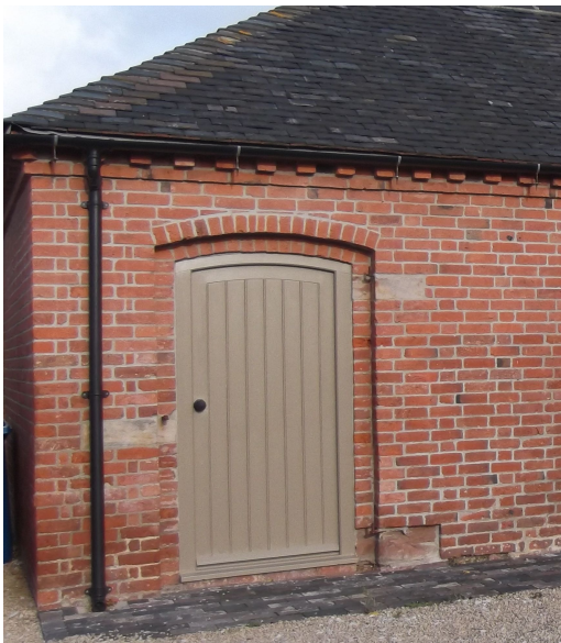
Picture B.9 A further example of repaired 'rise and fall' guttering
